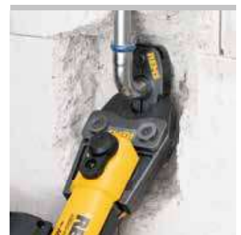
REMS pressing rings 45° (PR-2B) Patent EP 2 774 725
