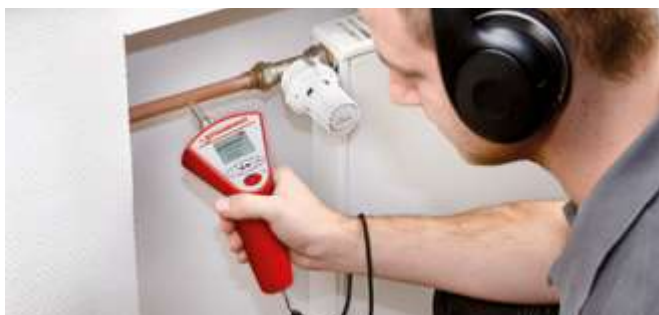
Acoustic leak detection of heating installations
